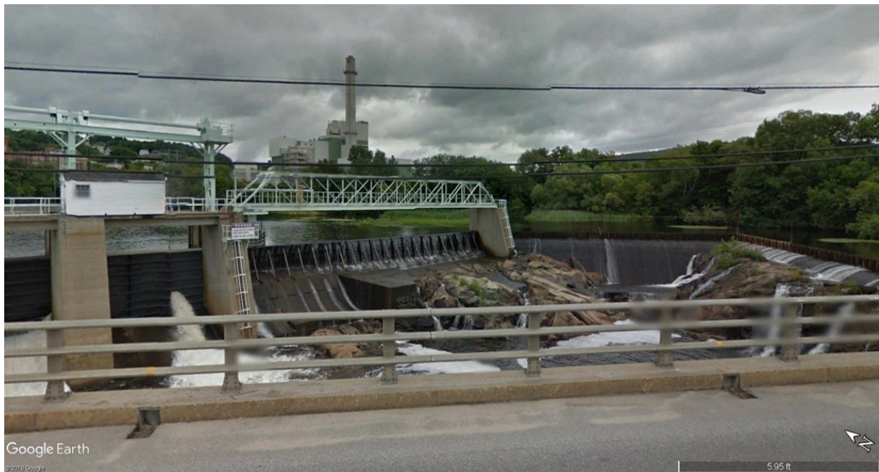
PHOTO 5-9 VIEW OF J. BRODIE SMITH DAM INCLUDING WASTE GATES, MINIMUM FLOW OPENING, AND SPILLWAY FROM THE MASON STREET BRIDGE.
