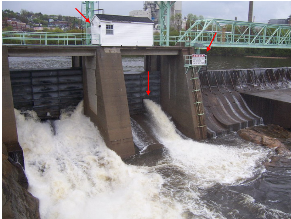
PHOTO 4-5 VIEW OF MINIMUM FLOW RELEASE ORIFICE AT J. BRODIE SMITH DAM. NOTE WARNING SIGN AND SIREN.
